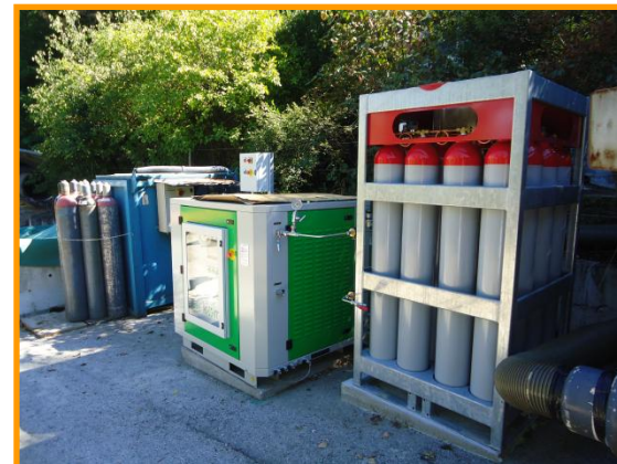
System for the biogas compression and storage
