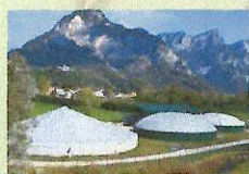
Biodigester of Villa Agneda (TN)
